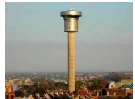
Harbour Control, Millers Point
