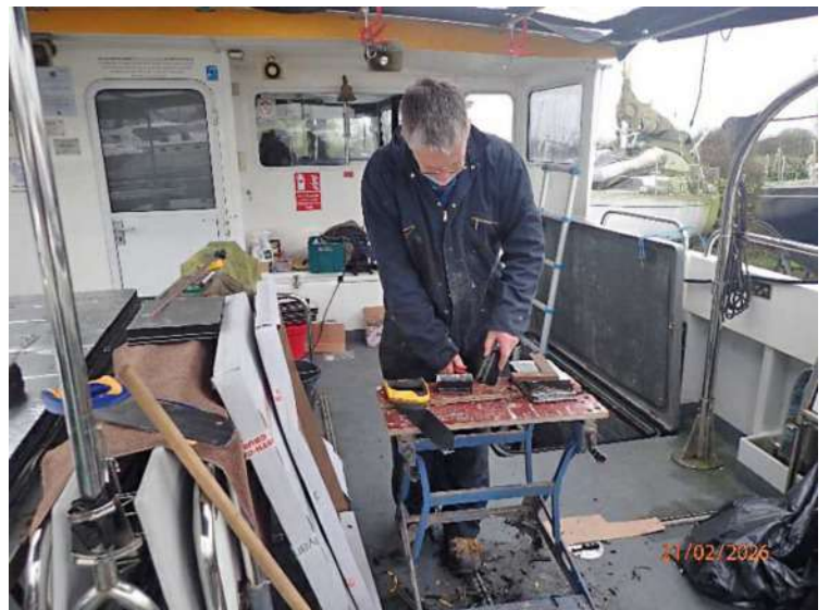
New insulation being fitted. Jeremy in charge of cutting!
