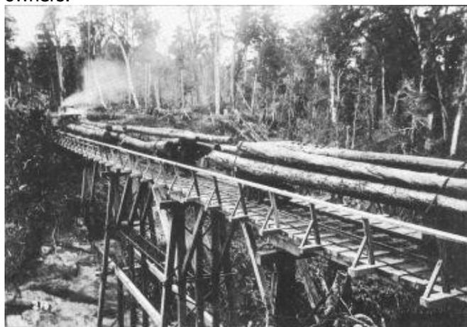
**Logs being transported along the tramway to the sawmill crossing one of the lesser viaducts**
