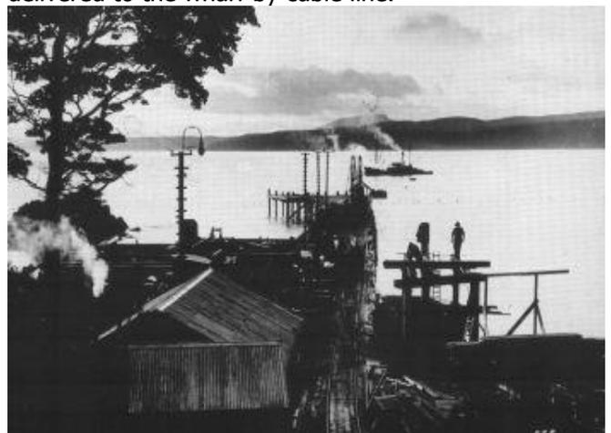
**Port Craig Wharf showing the ingenious cable loading system. The output at Port Craig broke New Zealand records. Port Craig was the largest and most modern mill in New Zealand at the this time.**
